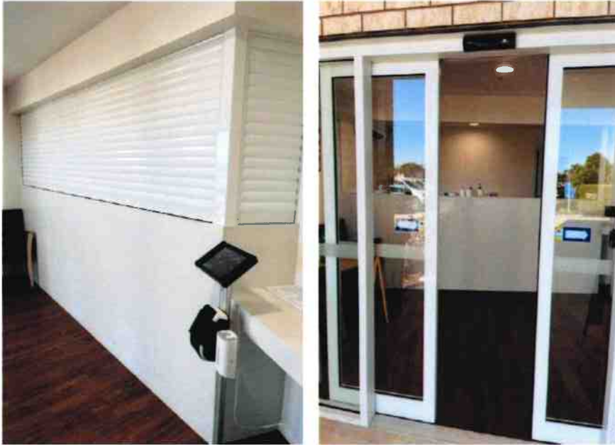
Front Entrance with Roller Shutters and Automatic Doors
