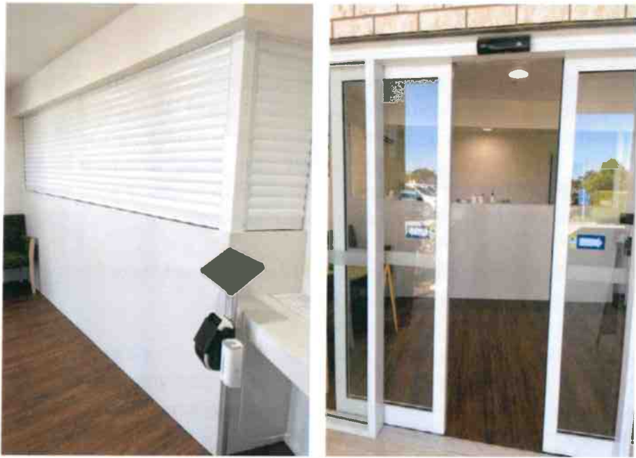
Front Entrance with Roller Shutters and Automatic Doors
